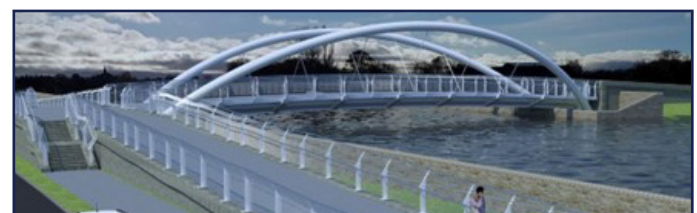
View of new Goosegreen Footbridge
