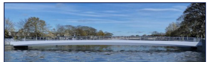
View of new Shorthope Street (Store) Footbridge
