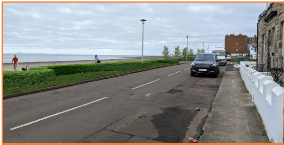
View of landscaping and planting at Fisherrow Promenade
