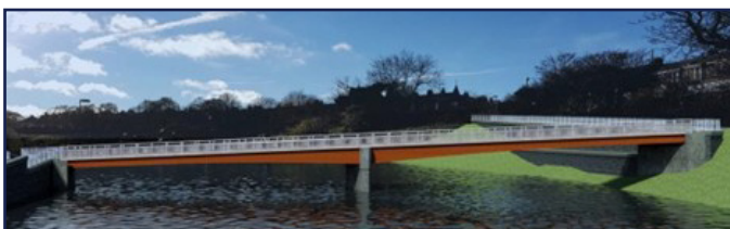
View of new Ivanhoe Footbridge
